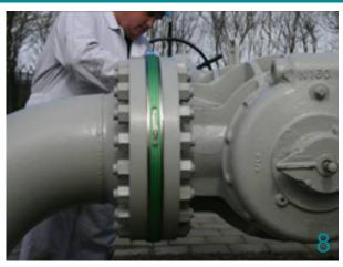
The rectangular cut in the ratchet strap enables tightening the clamp.
