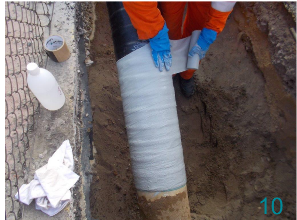
Work bottom to top.
