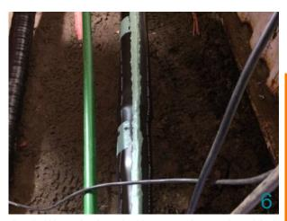
Apply Wrappingband without tension and avoid air enclosures. Press the Wrappingband in the pores of the substrate.
