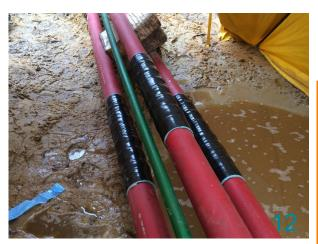
Apply Outerwrap with tension and avoid air enclosures. Overlap minimum 50%. Finish with 2 circumferential wraps and keep approx. 3mm Wrappingband exposed.
