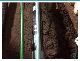
Apply Wrappingband without tension and avoid air enclosures.
