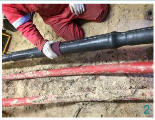
Prepare the entire casing incl. approx. 150mm of the high voltage cable.
