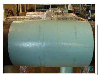
The overlaps of the straight wraps must not be in line with the previously applied straight wrap, their position should alternate.
