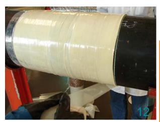
Outerglass Shield should overlap the factory applied coating approx. 100mm.
