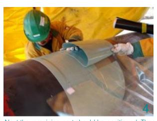
Next the remaining part should be positioned. Then remove the release liner and the Wrappingband has to be fixed to the surface. Avoid air inclusions.
