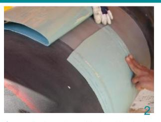
Start application at the 10 o'clock position. Apply Wrappingband with minimum tension and avoid air inclusions.
