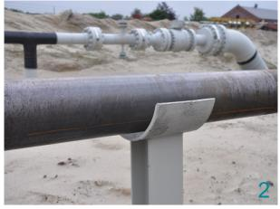
For the ease of application, lift the pipe at least 200mm.
