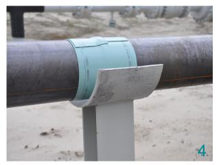
Apply Wrappingband with minimum tension and avoid air inclusions.
