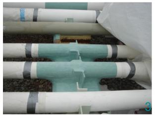
Apply Stopaq Basecoat over the entire support with a minimum overlap of 10mm on a previous applied strip Basecoat.
