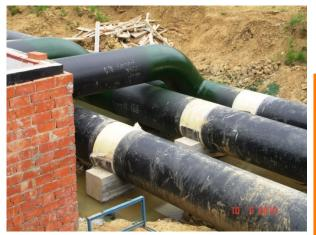
Pipe can be placed in the support after initial curing time of the Outerglass Shield XT. Polyester can be used as an alternative extra mechanical protection layer.
