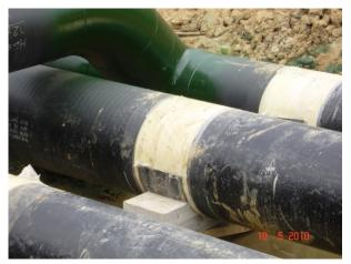
The coating performance will not be badly influenced when the compression foil remains on the Outerglass Shield XT.
