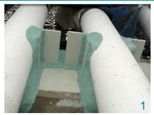
Ensure a proper surface preparation prior to the application. Apply Paste CZ in the sharp edges, under and around the pipe at the contact on the support.
