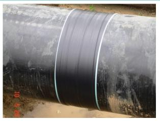
Keep 3mm of Wrappingband exposed at both ends.
