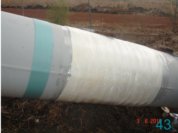
The coating performance will not be influenced when the compression foil is not removed.
