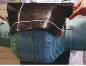
Width of the Geotextile should cover the complete area coated with Paste, but overlap on the Wrappingband should be avoided.
