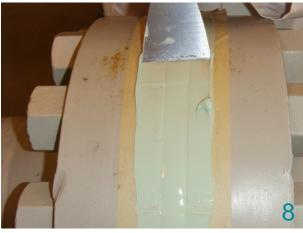
Prevent 4200 Filler from adhering to the surface of the flange.
