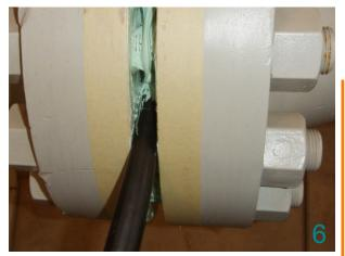
Fill the area between the flanges with the application tool and flexible nozzle. Work from inside out to prevent air inclusions.
