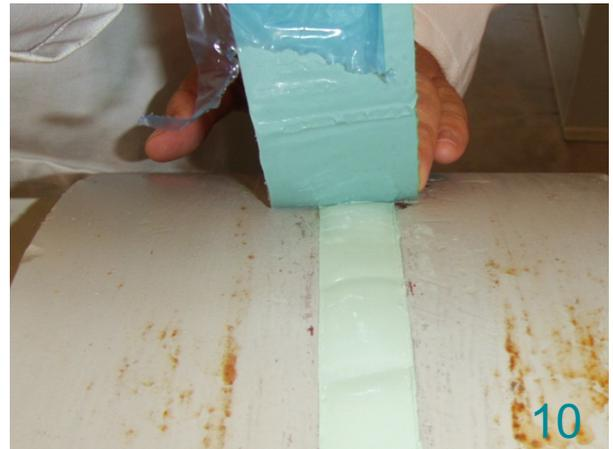
Wrappingband shall be applied without air entrapments. Fold the Wrappingband back into the Paste.
