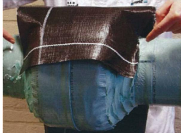
Width of the Geotextile should cover the complete area coated with Paste, but overlap on the Wrappingband should be avoided.
