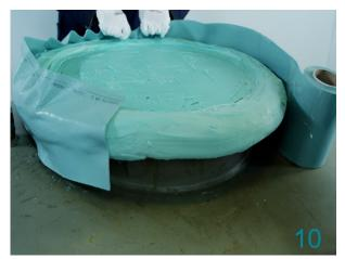
The Wrappingband will not adhere to the 4100 Putty. The width of the Wrappingband should be such that the bolts and nuts are covered.
