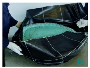
Put the geotextile around the manhole cover.
