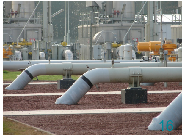
14 Paint the above ground part of the riser with a UV resistant topcoat to prevent discoloration of the Outerglass Shield XT.
