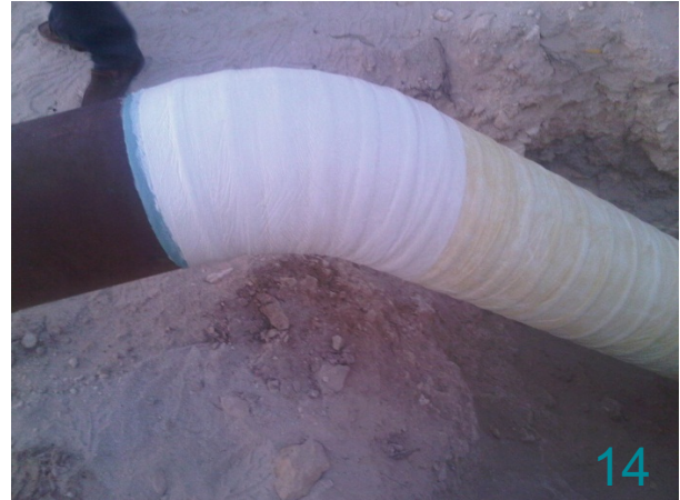
14 Paint the above ground part of the riser with a UV resistant topcoat to prevent discoloration of the Outerglass Shield XT.
