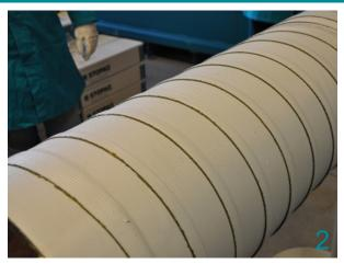
Start and finish with a straight circumferential wrap. Wrappingband CL shall be applied with tension.
