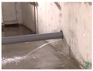
The sealing system can be applied while the duct is leaking.
