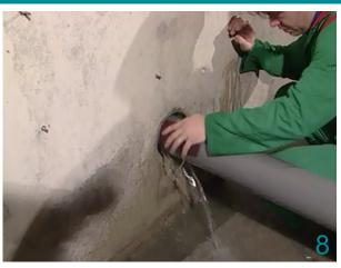
Adhesion can be improved when pipe and duct are pre-applied with 2100 Aquastop.
