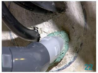
A cable can be removed from the duct with the same procedure. Remove the cable  $\rightarrow$  Apply 2100 Aquastop and Mortar WR or FR.
