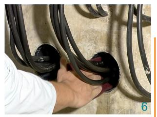
Adhesion can be improved when cables and duct are pre-applied with 2100 Aquastop.
