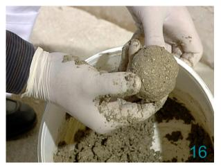
Mortar FR must be used in fire rated walls and floors. Check the malleability of the Mortar FR-WR by moulding the Mortar to a ball shape without falling apart.
